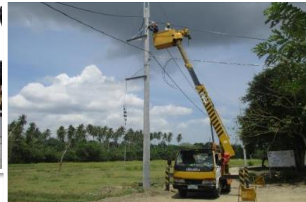
Primary and Secondary Line Stringing at Brgy. Del Valle, San Antonio, Quezon
