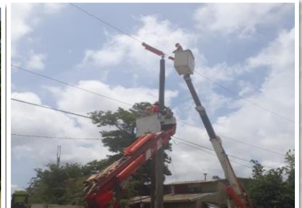
Pole Dressing at Sitio, Kabaisan, Brgy. Kulapi, Lucban, Quezon
