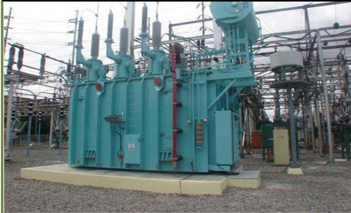
Replacement of Novaliches Power Transformer
