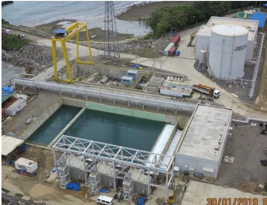
Aeration Pond, Electrical Control Building, Intake Structure & Water Treatment Area
