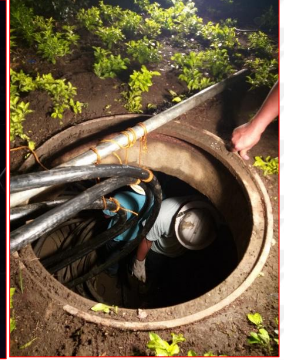
Splicing of underground cables
