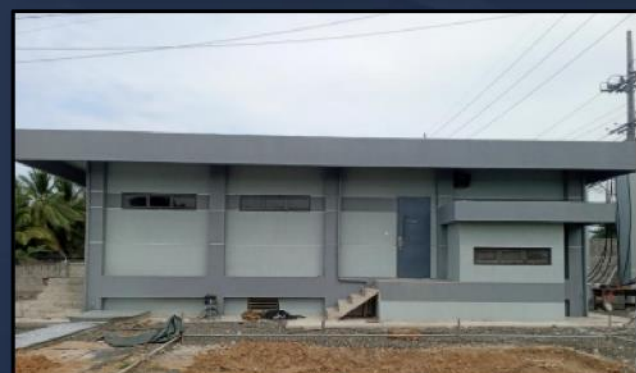
New Switchgear House
