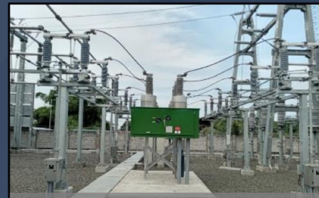
Breaker & Disconnect Switches
