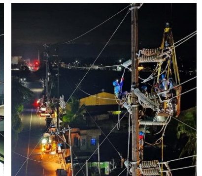
Uprating of Portion of Dila-Real 115 kV Line
