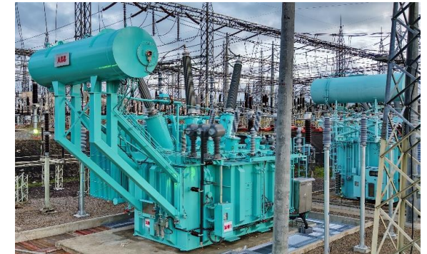
Upgrading to 300 MVA of 230 kV–115 kV Tayabas Power Transformer
