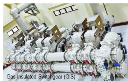
Gas-Insulated Switchgear
