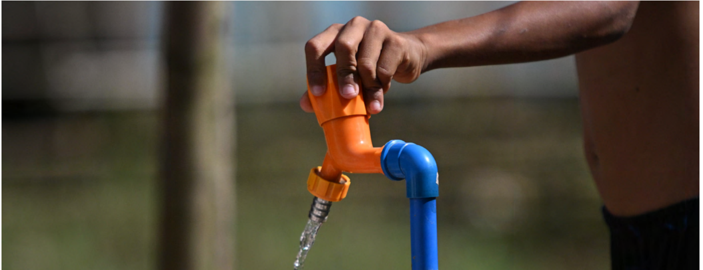
Water flows freely in Sitio Bulabog, Pilar, Sorsogon after OMF energized its water facility through solar electrification.
