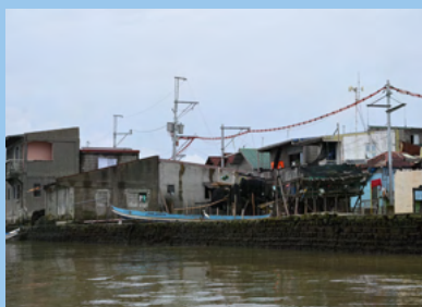
New power lines stretch across the waters of Hagonoy, Bulacan, delivering safe electricity to low-income fishing households through the Household Electrification Program.
