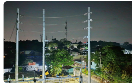
Construction of Parang-Marikina 115 kV Line
