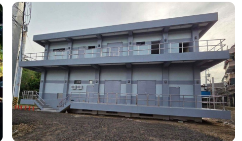
Construction of New Control House with Switchgear Room at Malabon Substation
