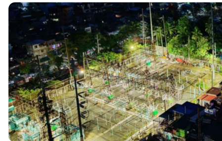
Uprating of 115 kV Power Circuit Breakers at North Port Substation
