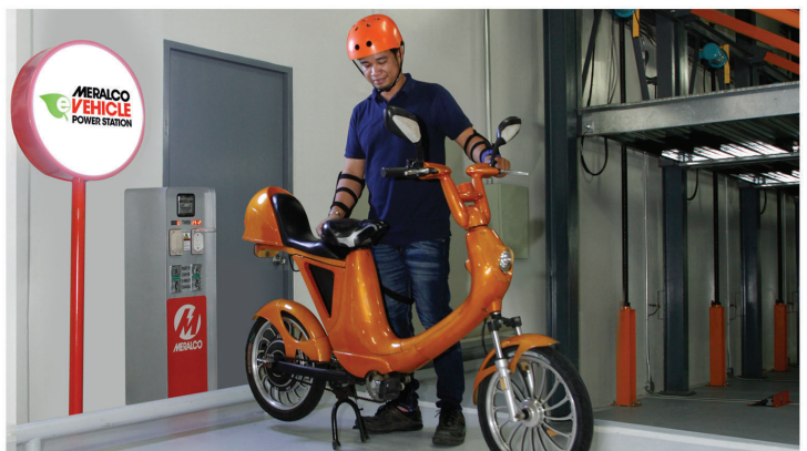
MServ licensed e-bike operator tests the newly-constructed EV charging station at Net Park.
