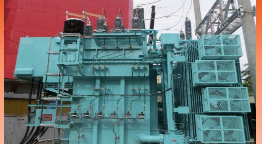
Replacement of Transformer Bank No. 2 at Mandaluyong Substation Completed Dec. 18, 2015
