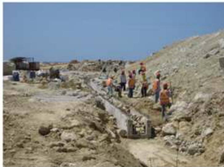
Toe drain (lower ditch) construction at Zone 2
