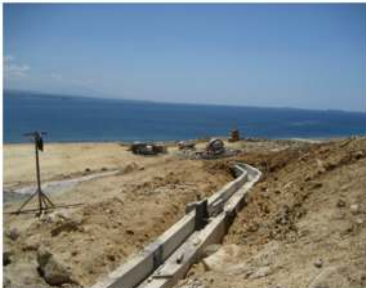
Completed head drain (upper ditch) construction at Zone 1
