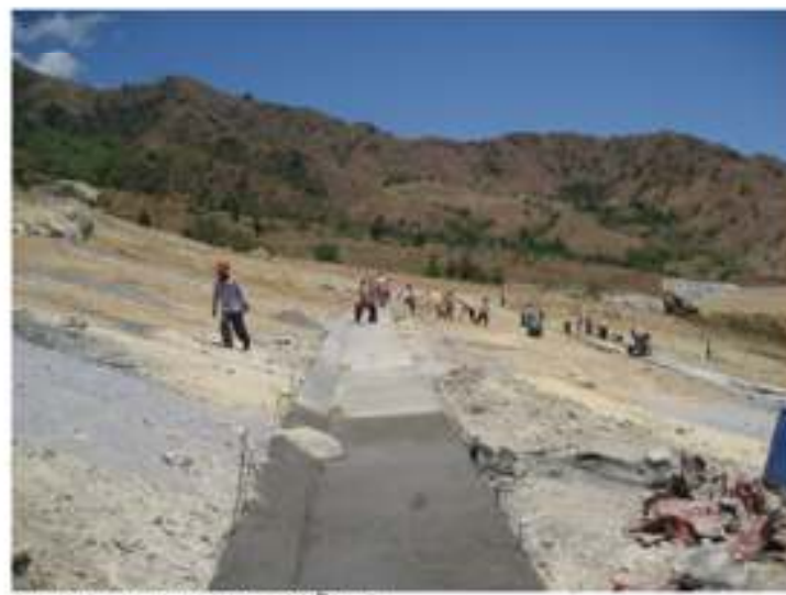
Berm drain construction at Zone 2 (4 th level)
