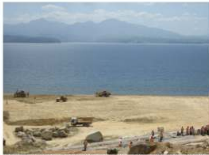
Spreading, leveling, grading and compaction of fill materials (coming from the trimming of area A-II slope) at areas A-II & III
