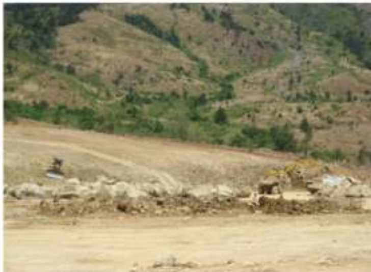
Trimming of slope at Zone 3, and hauling of fill materials & boulders
