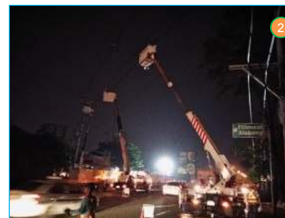
Sept. 30 to Oct. 1, 2015 - Relocation of Distribution lines along Osmeña Hi-way cor. Quirino Ave.
