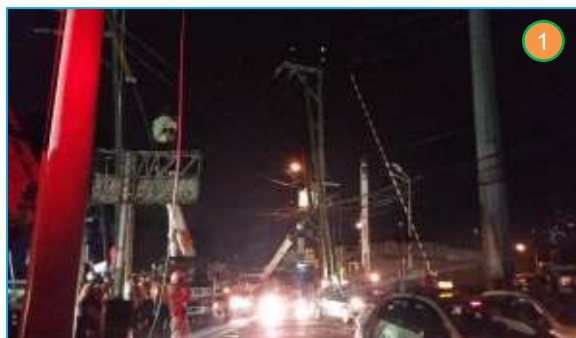
Aug. 31 to Sept. 1, 2015 - Relocation of distribution lines along P. Ocampo, Manila
