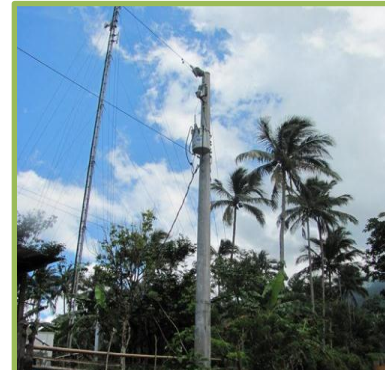
Newly installed concrete pole & 20KV distribution transformer
